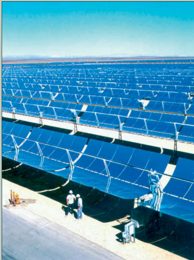
Rows of parabolic mirrors concentrate sunlight on the tubes in the middle. Oil inside the tubes, which is heated by the concentrated sunlight, is used to generate electric power.
